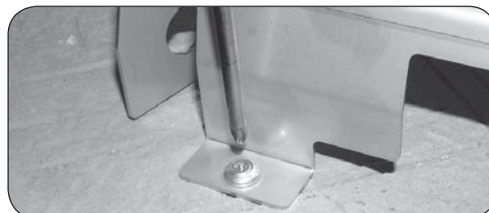
Fig. 15-2 Fasten hammer screws
