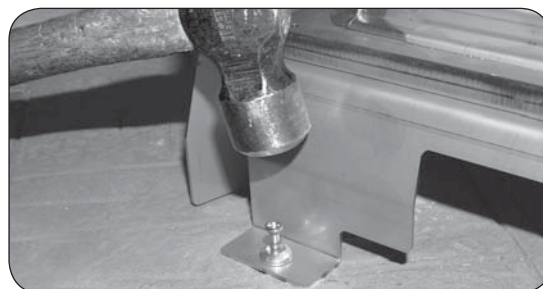
Fig. 15-3 Install hammer screws
