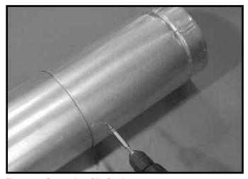
Figure 7.4 Screws into Slip Section
