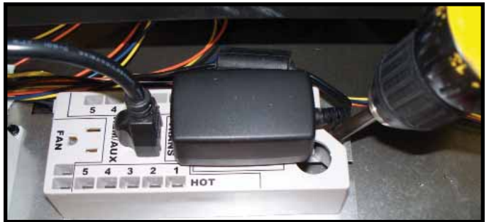
Figure 8.2 Junction Box Detail
