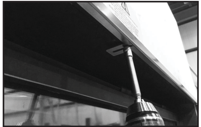
Figure 10.5. Install Trim Ring
