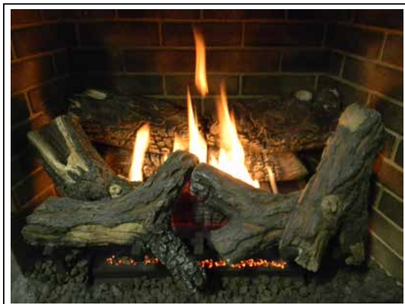
Figure 36 - Burner Flame Appearance
