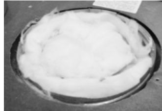
Step 3: Remove insulation from inside flue pipe.
