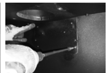
Step 8: Remove the 4 screws around the rear vent and use to Re-install block off plate and gasket over the rear vent flue.
